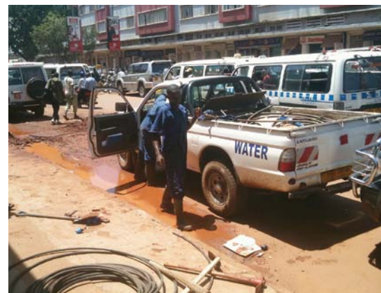
Leak-repair crew in Kampala, Uganda.
