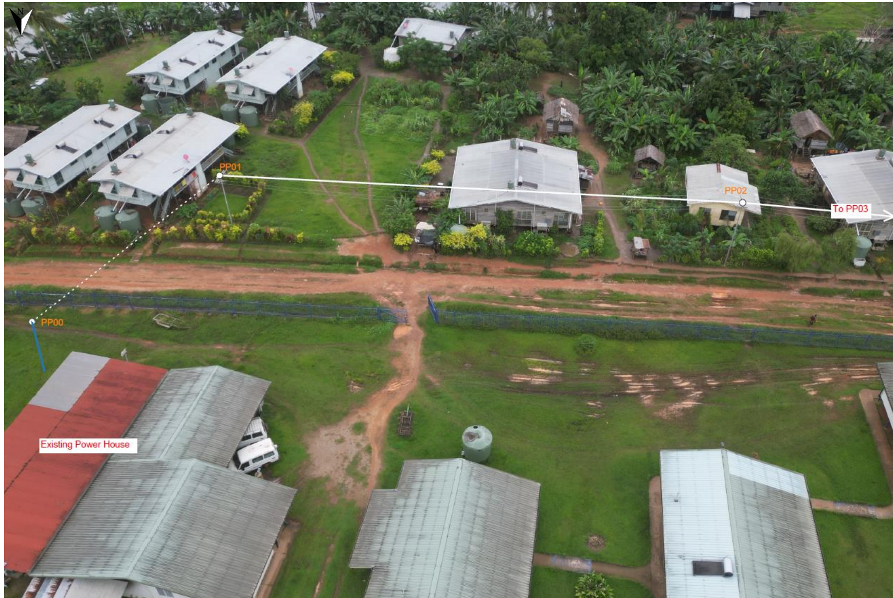
Figure 5. Power poles PP01, PP02 and PP03 that need to be disconnected from the town grid and connected to the Hospital grid
