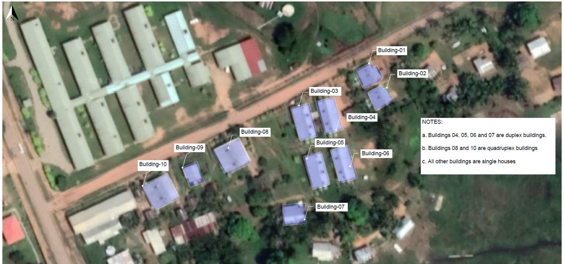
Figure 3. Balimo Hospital ten staff houses that are currently connected to the town grid and need to be connected to the Hospital grid
