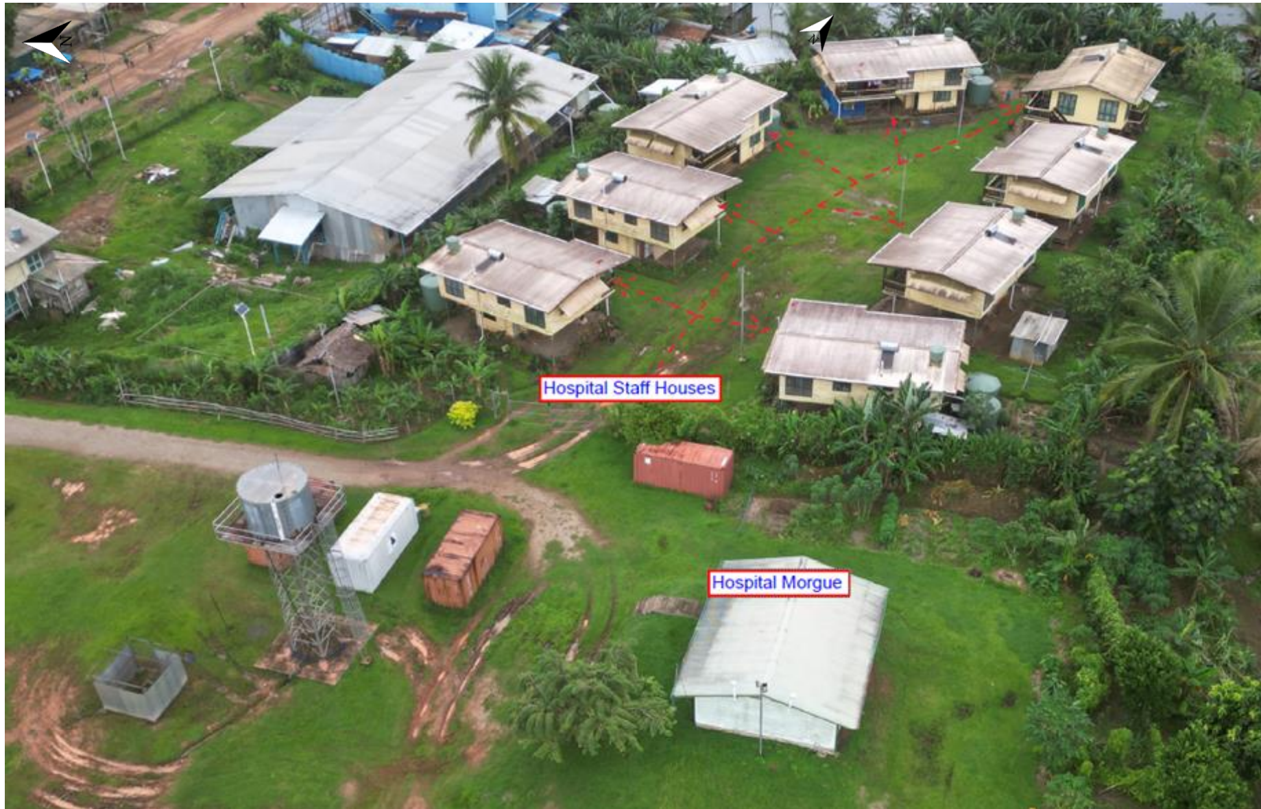
Figure 6. The eight staff houses currently connected to the Hospital grid
