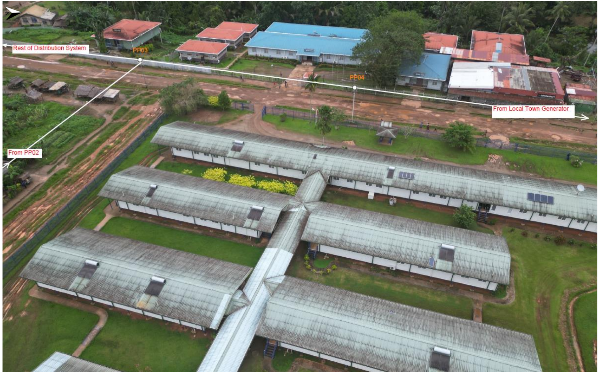
Figure 4. Power poles currently connected to the town grid around the Hospital compound
