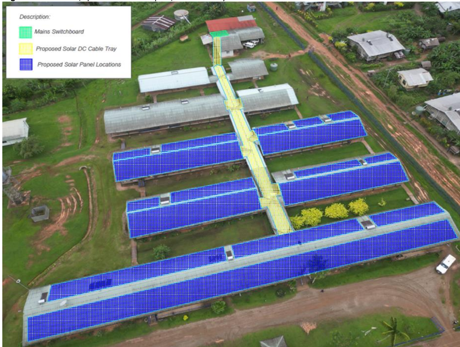
Figure 7. Available rooftops at the Balimo Hospital for solar PV array
