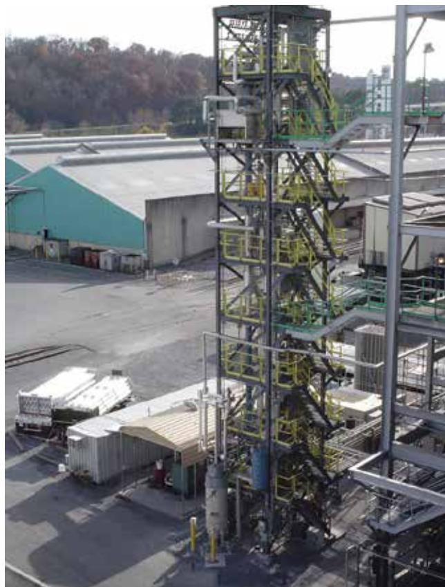
Figure 5. WDP Pilot Plant
